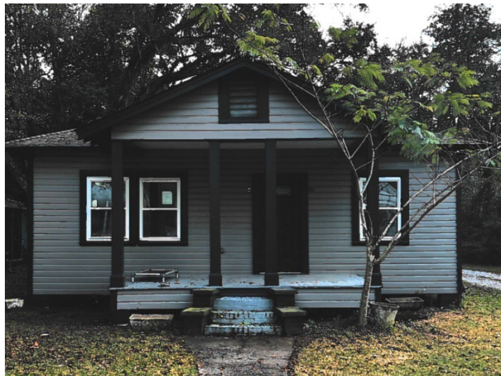
Figure 2. 707 W Hall Avenue
