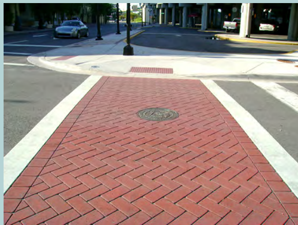
This pedestrian crosswalk's brick paving and concrete banding are not only attractive, but drivers can feel it under their tires to be reminded of the presence of pedestrians. It is recommended for both Front Street and Fremaux Avenue.
