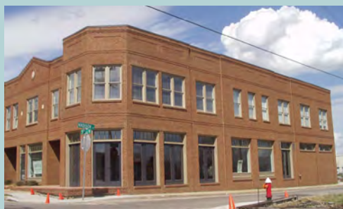
This newly-developed mixed use building would fit nicely into many historic areas. Primary design features include groundfloor storefront windows, vertically-oriented upper floor windows, a flat roof visually screened with a parapet facade, traditional building materials, and varied facade massing.
