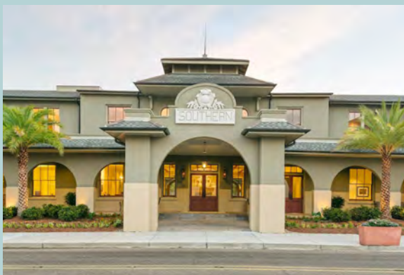
The Southern Hotel opened in 2014 in Downtown Covington, Louisiana. After sitting vacant for many years, this historic 1907 hotel was rehabilitated with the help of federal and state investment tax credits for historic rehabilitation. As a new anchor to Downtown Covington, it features 40 rooms and a white cloth restaurant.
