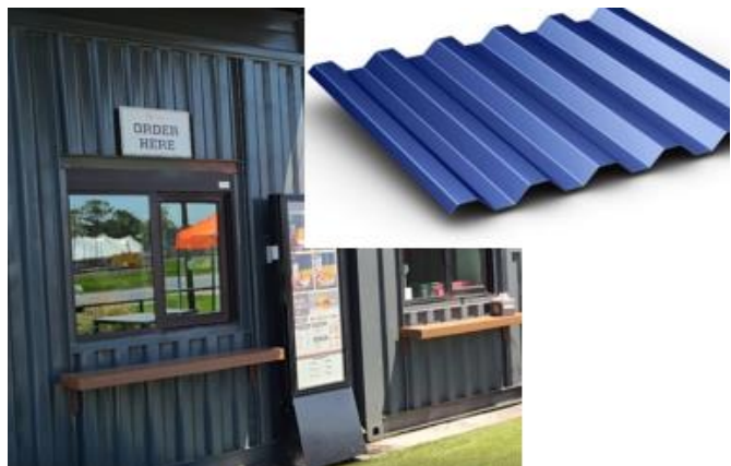
Figure 5. Sample Materials – Metal siding (Baton Rouge Location)
