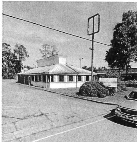
Figure 2. Existing property condition
