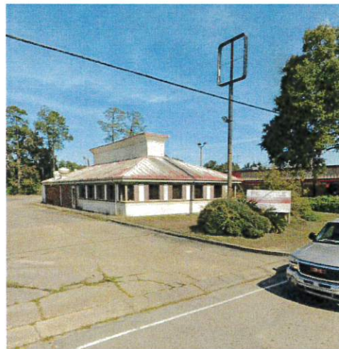
Figure 2. Existing property condition
