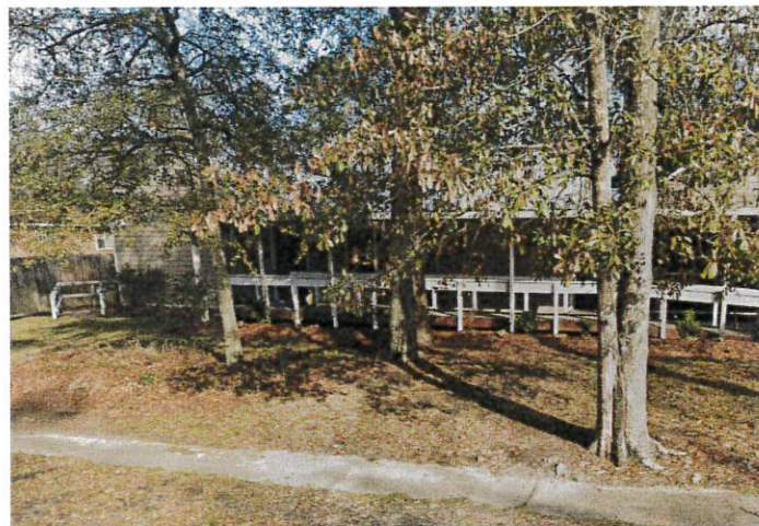
Figure 2. Existing exterior of building
