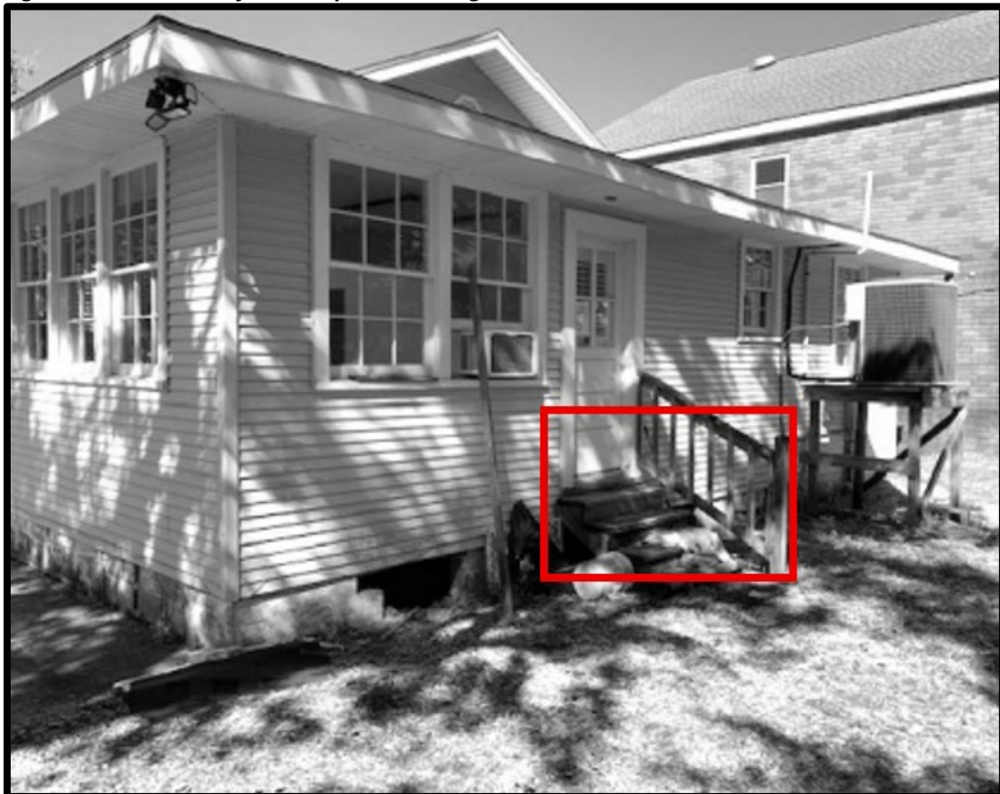
Figure 3.d. Removal of rear steps and railing
