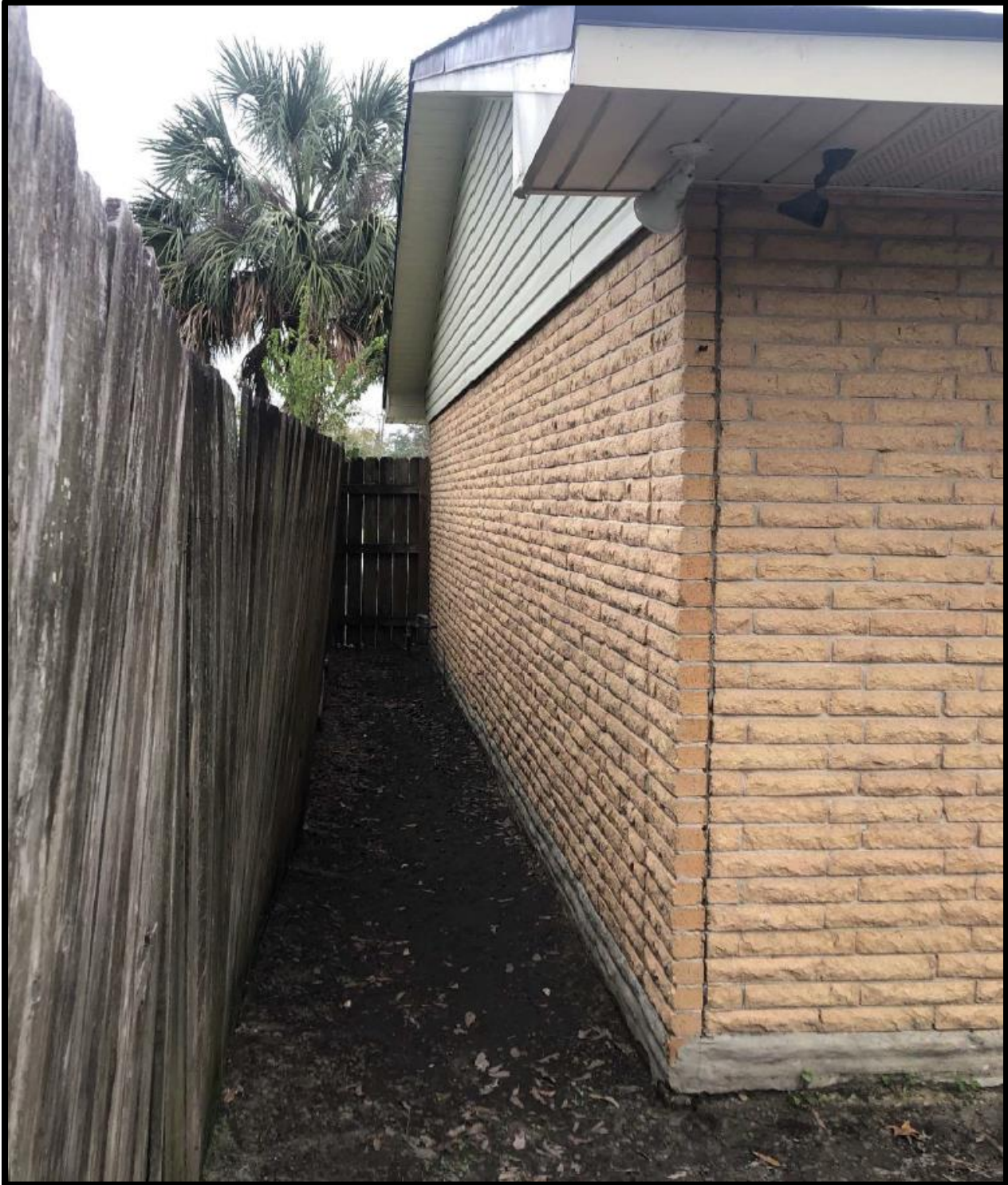
Right Side Yard – setback at 5.1 feet (fence is not on property line)
