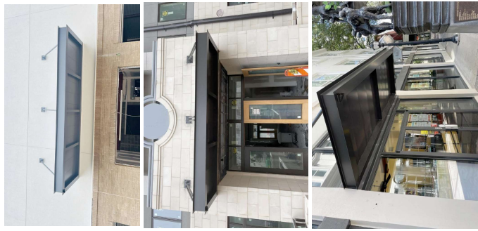
5 Example Images Of Aluminum Canopy Style & Color A300 Scale: None Note: Manufacturer: Skyscape Architectural Canopies, Color: Powder Coated Black
