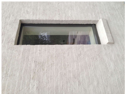
2 Example Image Of Proposed Sacked/Smear'd Brick Finish A300 Scale: None Note: Sacked/Smear'd Brick Finish To Be Painted Sat White
