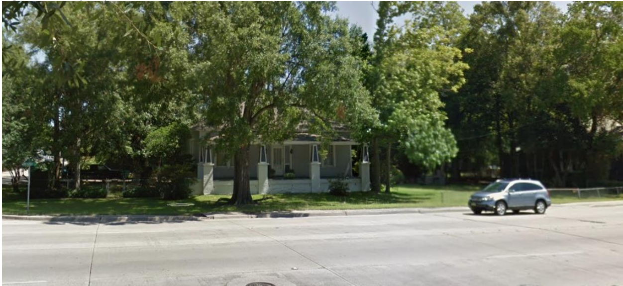
Figure 2: Property Current Conditions
