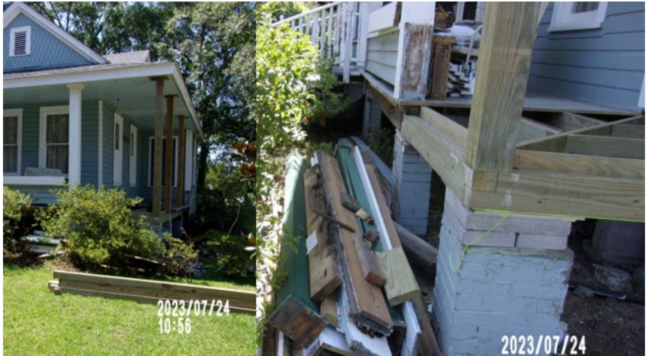
Figure 3. Repair of rotted wood at front porch
