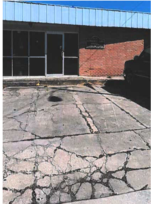
Figure 7. New Paving Area
