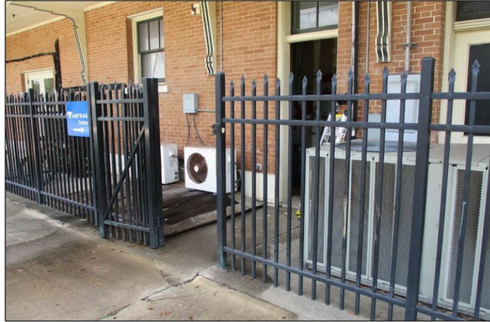
Figure 6: Existing Ornamental Fence.
