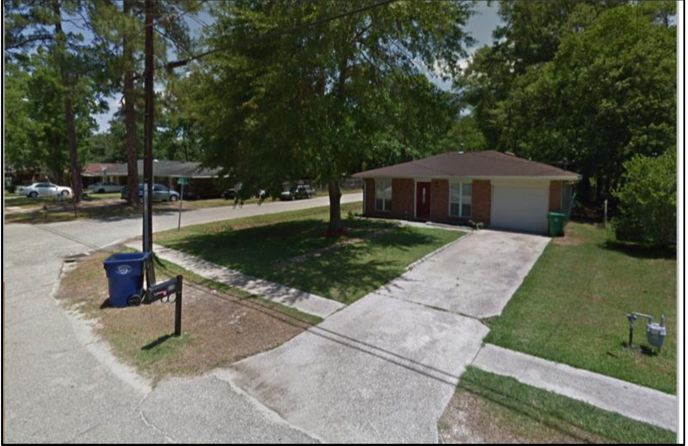
Figure 2: 806 Pine Tree St Street View Pre Elevation
