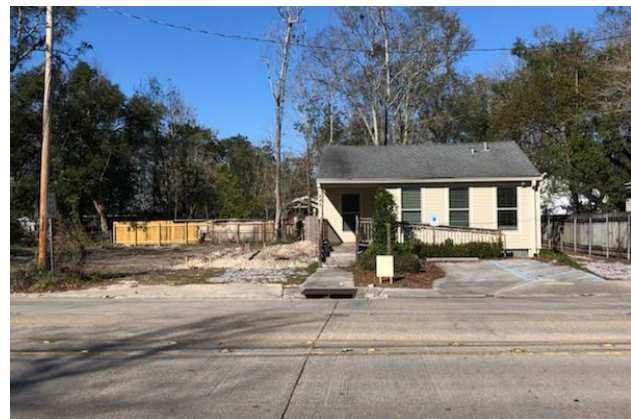
Figure 2. Property Current Conditions
